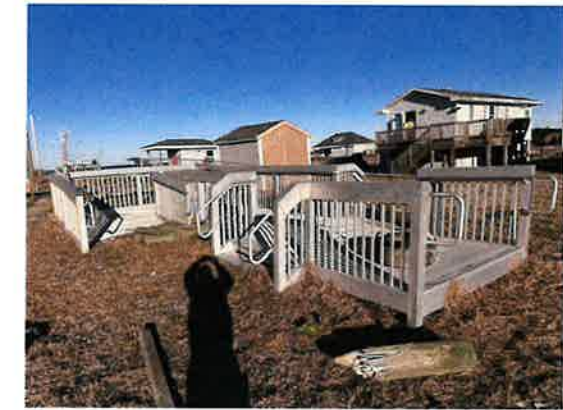
PHOTO 1 - RAMP AT SOUTHDOCK
